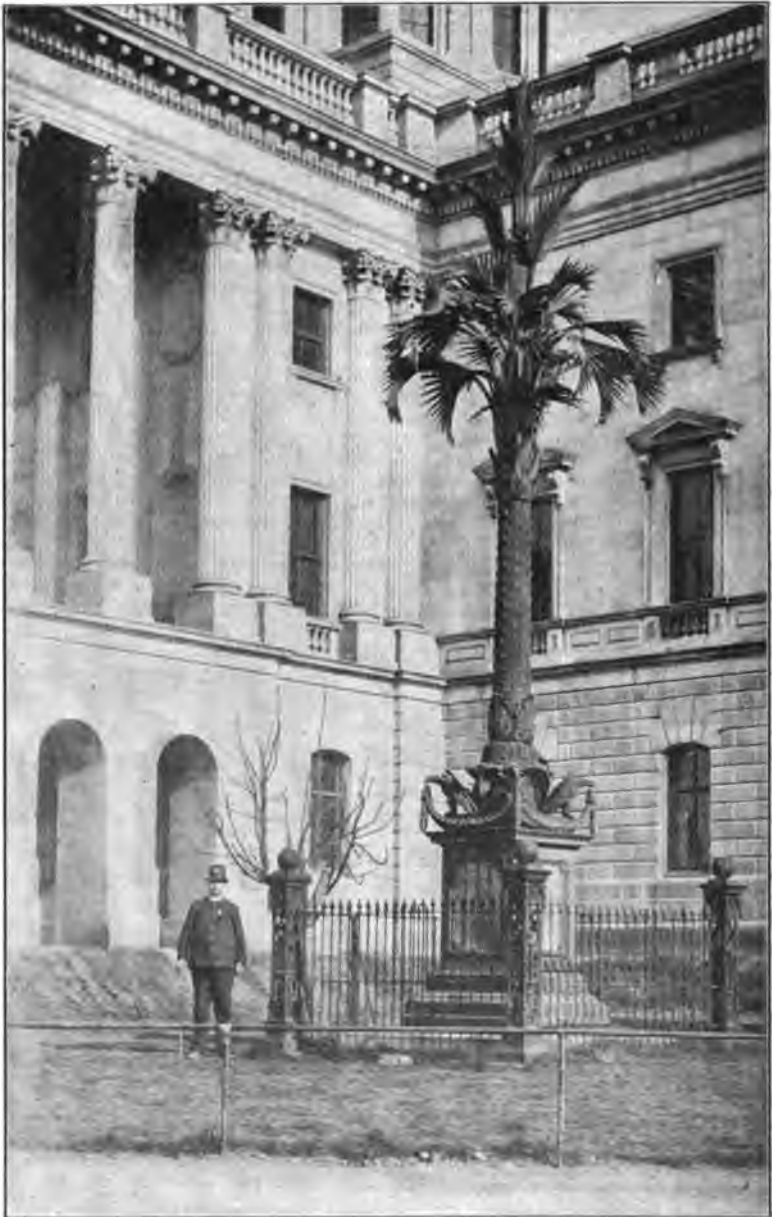
MONOLITH COLUMNS—22 TONS EACH. SOUTH CAROLINA GRANITE.
